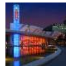
Metal Tensile Structure
