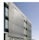
Parking Garage Facade, Ventilation System
